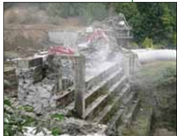
Elwha gravity dam removal.
