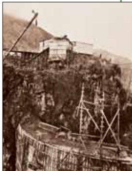
Construction of the Glines Canyon Dam, circa 1925.
