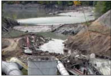
Working below the safety of the log boom.
