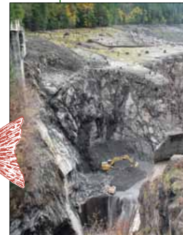
Glines Canyon Dam removal progresses.
