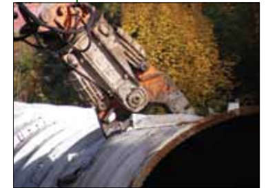
Removal of penstocks.
