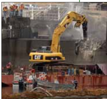
Glines Canyon Dam demolition begins.
