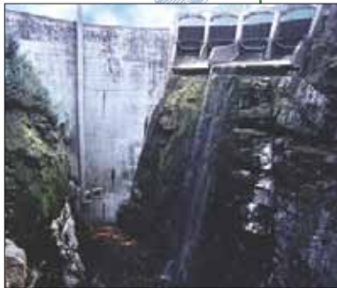
Glines Canyon Dam
