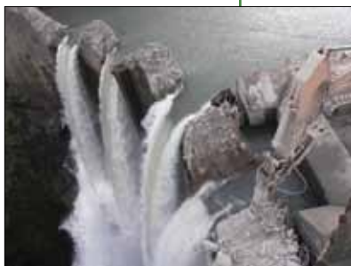
Notching Glines Canyon Dam.
