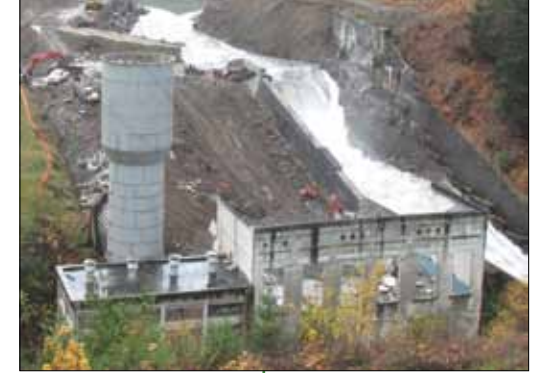
Elwha Powerhouse demolition, 2011.
