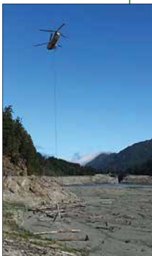
Helicopter transporting woody debris to reservoir bed.
