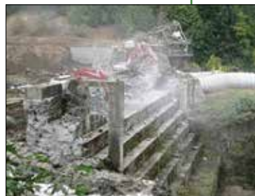
Elwha gravity dam removal.
