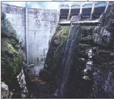
Glines Canyon Dam
