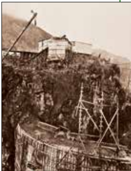
Construction of the Glines Canyon Dam, circa 1925.
