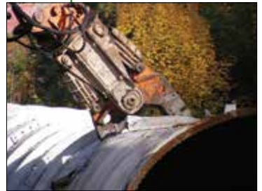
Removal of penstocks
