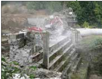
Elwha gravity dam removal
