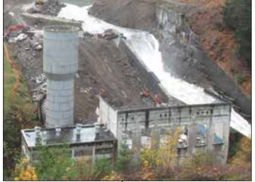
Elwha Powerhouse demolition, 2011
