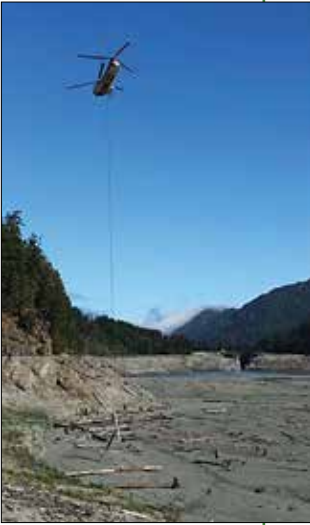
Helicopter transporting woody debris to reservoir bed
