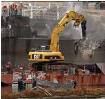
Glines Canyon Dam demolition begins.
