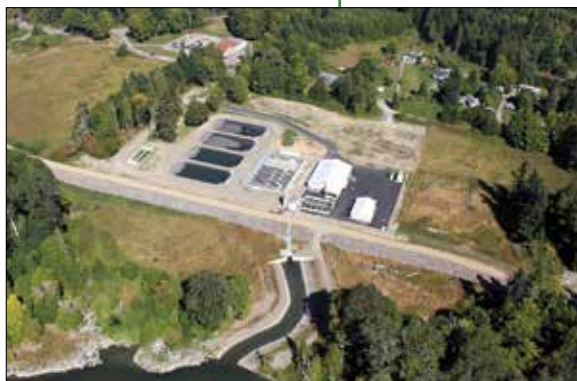
An aerial view of the new Elwha River hatchery, 2011
