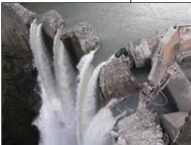
Notching Glines Canyon Dam.
