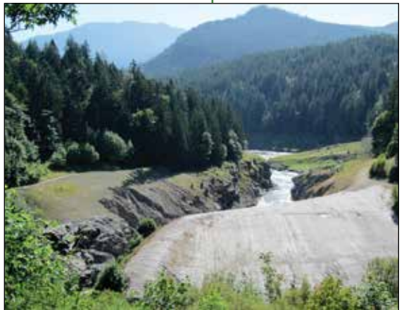
Former site of the Elwha Dam, circa May 2012.
